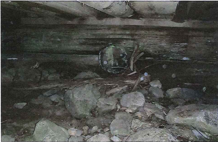
CK2284 Right Abutment
